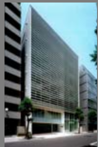
Head Office Annex The center for systems technical support
